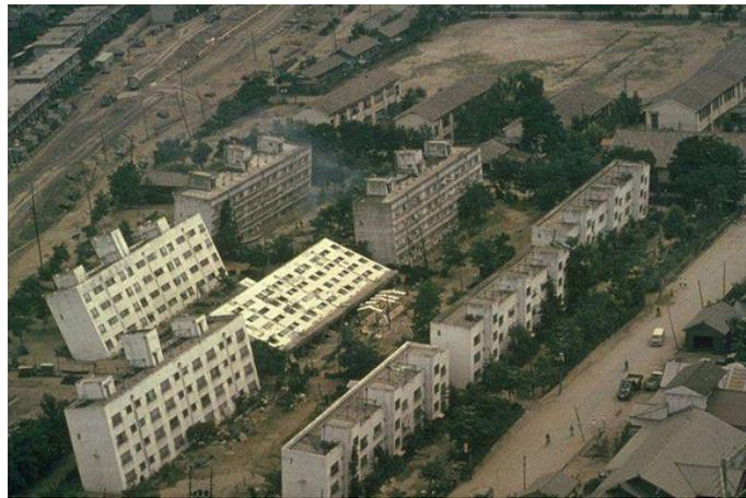
Figure 1.1.: Structural Collapse during 1964 Niigata Earthquake [1]
